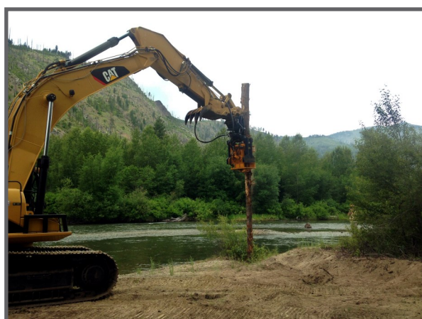
Pile driving technology, a proposed method for installing engineered logjams
