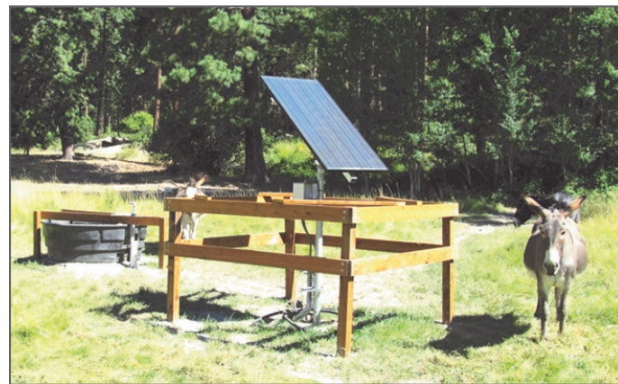
Completed solar-powered stock watering facility at Tyee Ranch in the Entiat watershed
