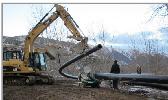
Welding and installation of the HDPE pipeline near Sunnyslope
