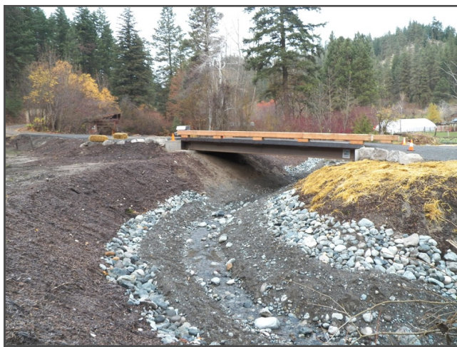
New steel bridge on Freund Creek that replaced an old culvert that had become a fish passage barrier
