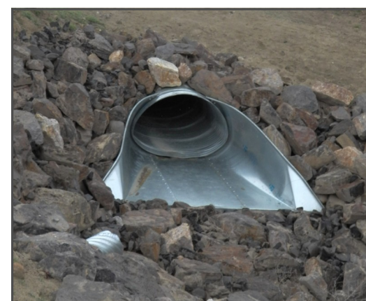
A large culvert makes it easier for debris to escape. Large rock around it will prevent erosion and help direct storm water runoff
