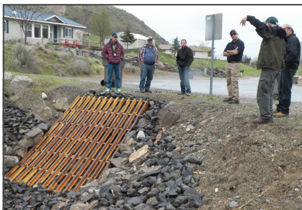
A re-purposed cattle guard is used to keep existing trash and debris out of culverts
