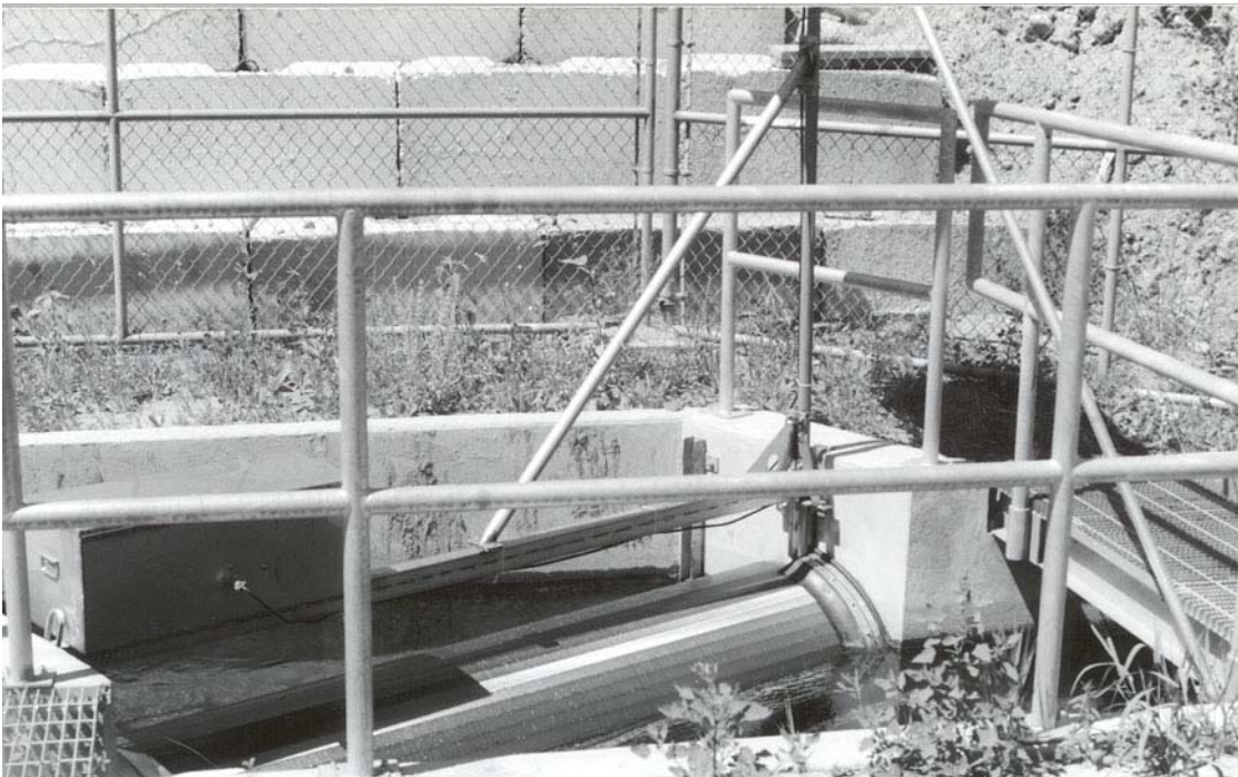
Figure 3-13. Close-up view Hanan-Detwiler fish screen.
