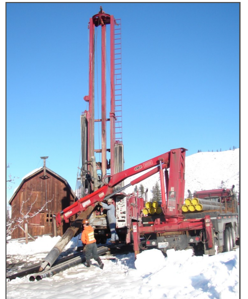
Drilling for surface to well conversion
